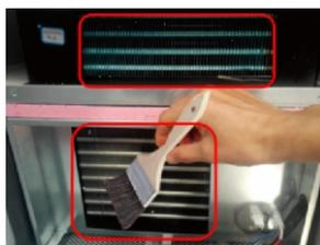
6. After cleaning is completed, close the baffle and tighten it with screws.
